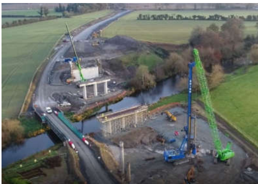
Construction of new bridge under the Dublin-Cork Railway Line, Easter 2018.
